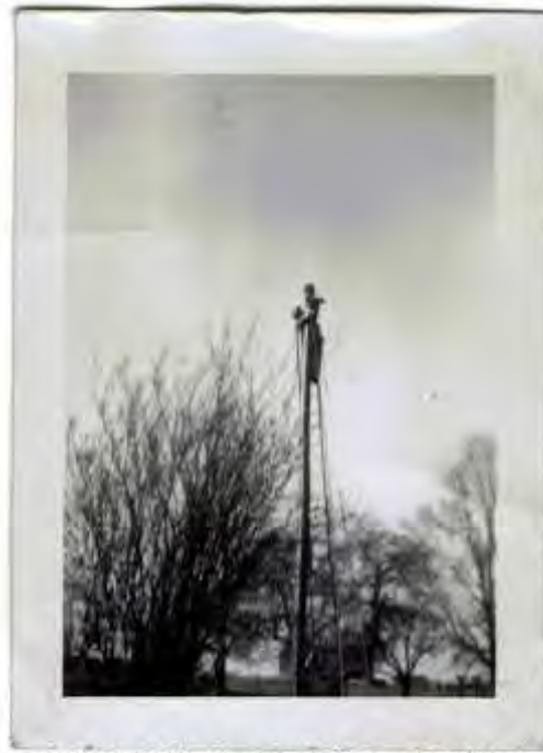
ph1311(1) Archie White 15-16ei. Installing hydro 1948 labelled "Clarence"
