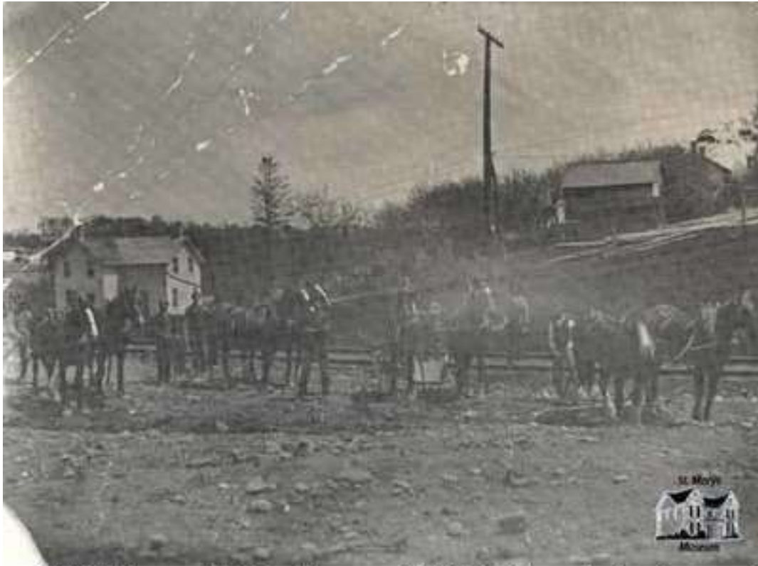
ph1903 Rosetta Fulcher Horton 60-61fak. House in background Building the Grand Trunk Station 1907 (St Marys Archive collection)
