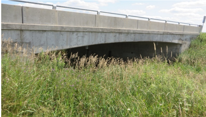
Wickie Bridge Structure 135018 - Perth Road 135 BCI – 54 (Fair)
