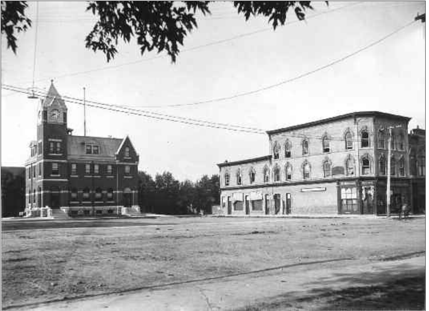
1042 A southwesterly view of Mitchell's market square, on the southwest corner of Ontario Road and St. Andrew Street soon after construction of the town's new post office and customs building was completed, in 1911. To the right is the start of the south side of the town's main business block, between St. Andrew and St. George streets.
