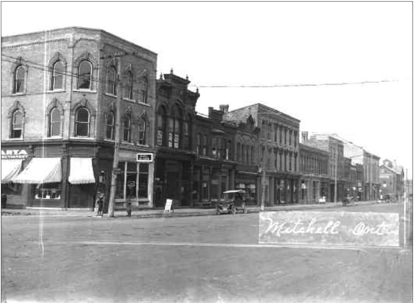
1025 A southwesterly view of the south side of Mitchell's main business block, between St. Andrew and George streets in the early 1900s. From the left: John McCutcheon's confectionery shop; the Mitchell Restaurant and ice cream parlour; the T. S. Ford general merchandise store; Dr. Robert McGill's dental office; and a boots and shoes outlet.
