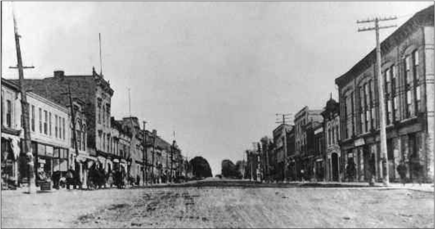
1032 A westerly view of Mitchell's main business block (Ontario Road), from its intersection with St. George Street. On the extreme left is Mike Durkin's grocery store. On the extreme right is the opera house that was built in the 1880s by Henry James. This photo appears to have been used as a poster or for the cover of a book or booklet.
