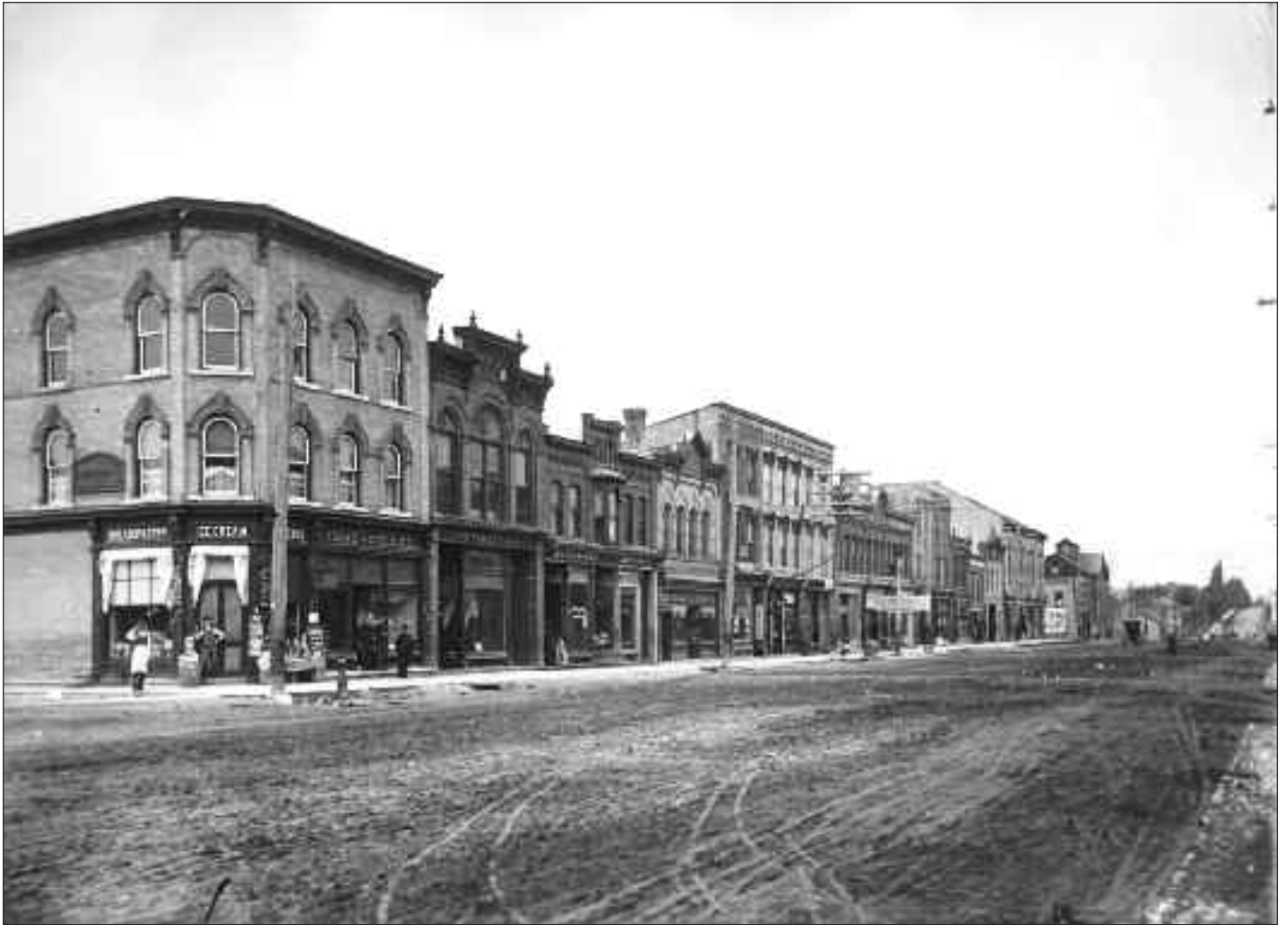
1024 A southwesterly view of the south side of Mitchell's main business block, between St. Andrew and George streets in about 1900. From the left: Isaac Hord's dry goods store, with Dr. Robert McGill's dental office; the T. S. Ford general merchandise store; the Middlemiss and Rankin hardware and tinsmith shop; a boot and shoe shop; Thomas Coppin's tailor shop; and the Burgess photography shop.
